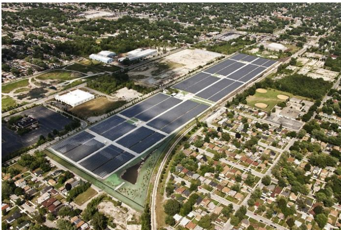
Figure 4: Exelon City Solar is a 10-megawatt solar installation located on a 41-acre brownfield in Chicago's West Pullman neighborhood.
