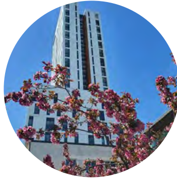
Daphne Cockwell Complex LEED GOLD V3
