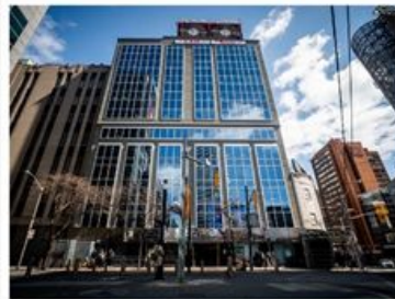
TMU will take possession of 277 Victoria Street in 2025 and is planning renovations to transform the space into an innovative facility for the Lincoln Alexander School of Law. Photo by Jae Yang.
