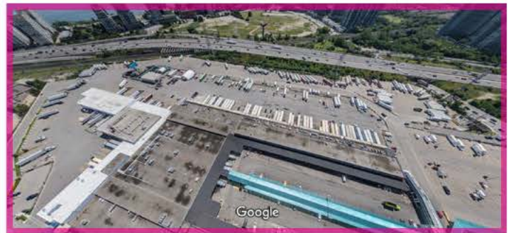
6 Aerial view of Ontario Food Terminal.
