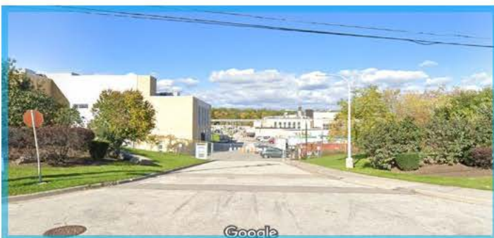
7 Entrance to the Humber Wastewater Treatment Plant from the Queensway.
