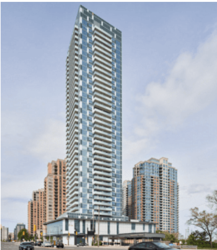
Figure 57: 5249 Dundas Street W
