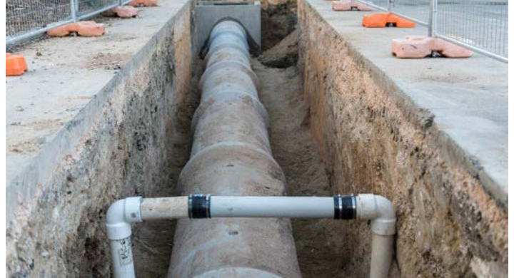
Figure 21: Illustrative Storm Water Pipeline (Wade, n.d.)
